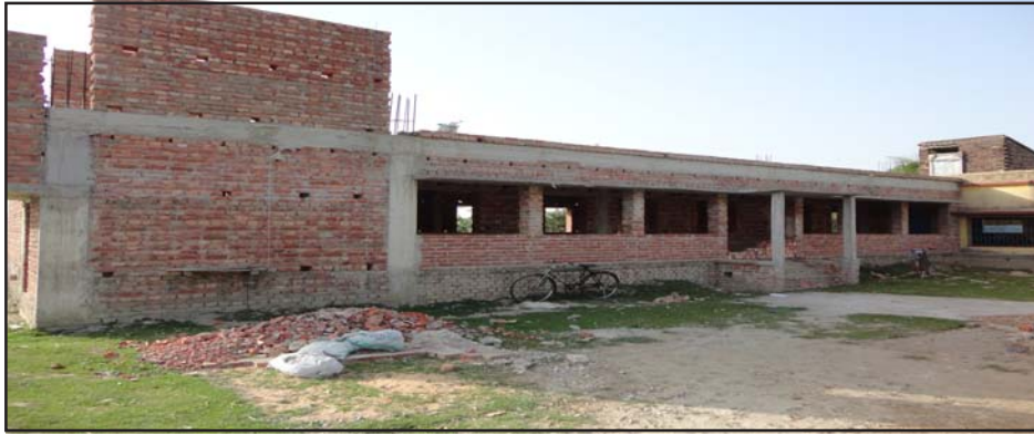
Under Construction of Vocational Training Centre for DMS
